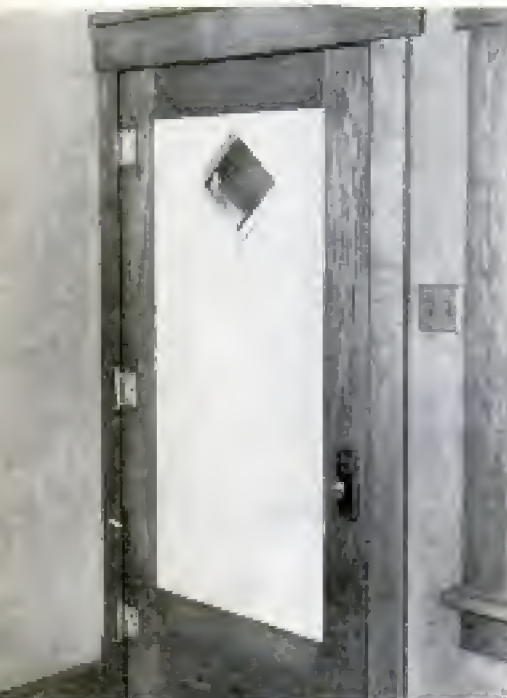
Above, assembly before refinishing. Below, door is filled, sanded, pointed white
